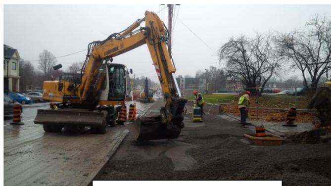
*Preparation of granular base for the temporary sidewalk.*
