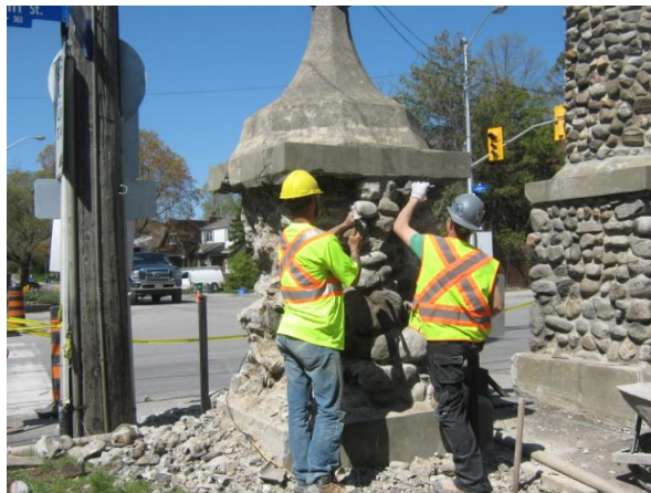
Removal of stone facing of the Brantwood Place Gates
