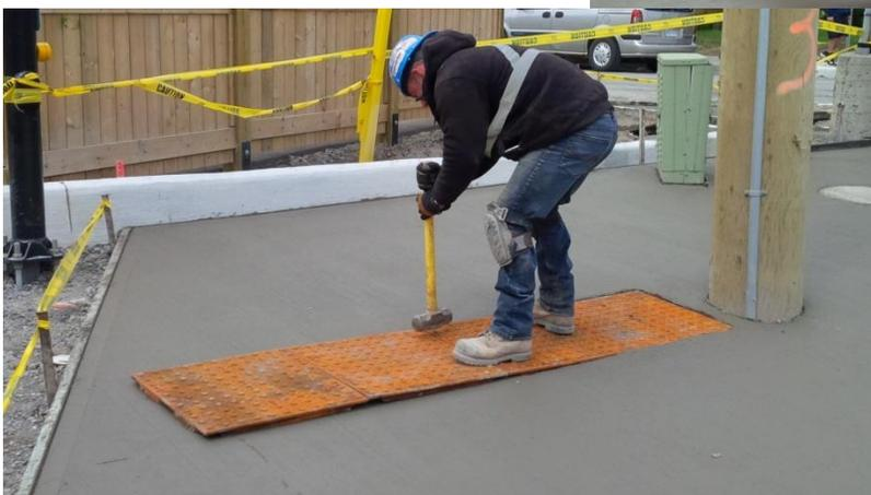
*Installation of TWSI in fresh concrete.*
