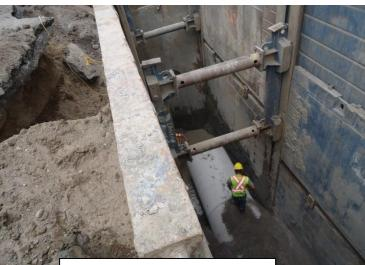
Installation of the 1,200mm diameter storm sewer by open cut (approximately 6m deep).
