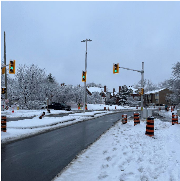
Photo 3: New Traffic Signals installed at 417 Onramp on Greenfield (December 2023)
