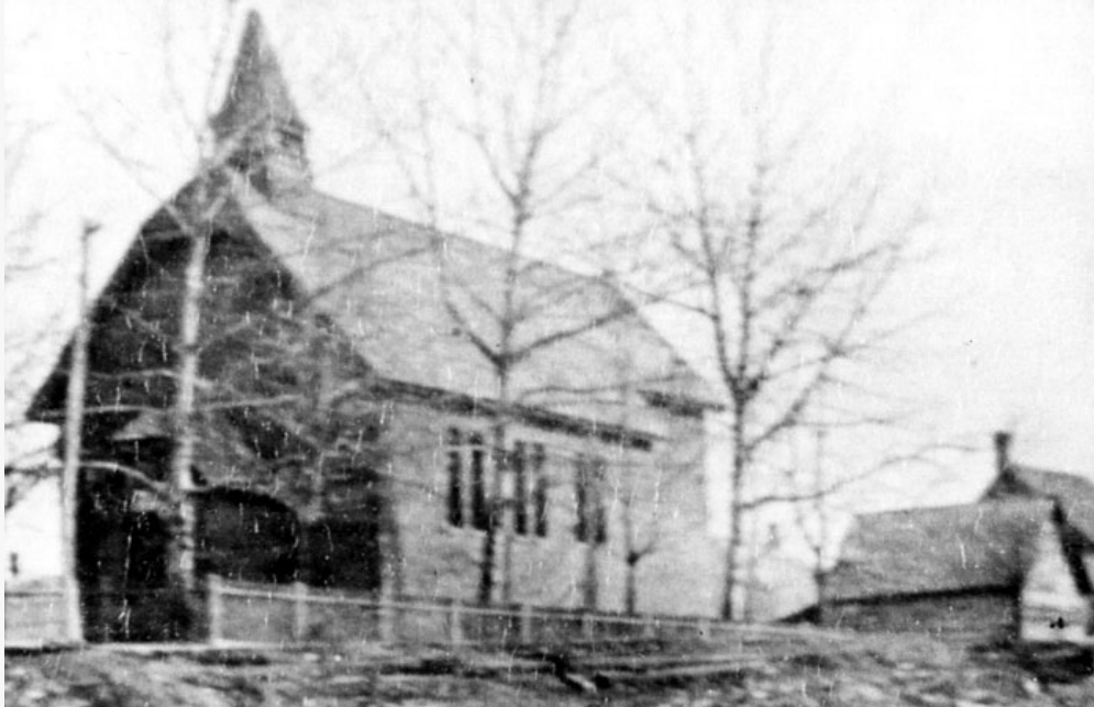
Trinity Anglican Church at Main and Echo Drive - c1890 The oldest church in Ottawa East and still standing
